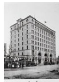
Tokyo Tatemono Building (former Tokyo Tatemono Headquarters Building)
