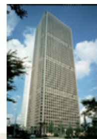
Shinjuku Center Building
