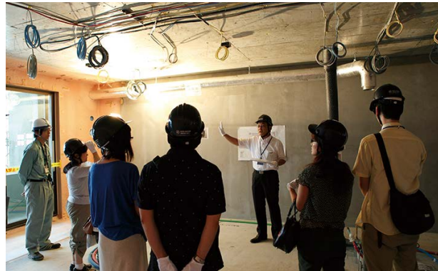
On-site Tour of Framework and Concrete Walls
