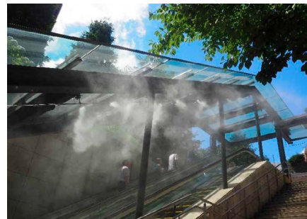
Fine mist decreases the ambient temperature from three to five degrees Celsius without passers by or things nearby getting wet.
