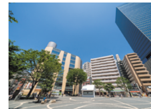
Naka-Ikebukuro Park (after renovation) is positioned as a temporary evacuation site for use in the event of a disaster.
