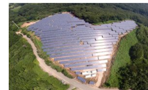
Hatoyama Solar Power Plant
